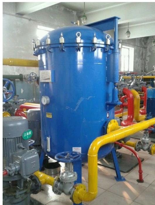
**DF60 Diesel Purification Filter** is being used to remove impurities, colloid and water. The pollutants (mostly exquisite colloid and water) need to be discharged from drain valve every week, and the filter was back-washing automatically every day. The capacity is 300 tons daily, and the service life will be 2~3 years.
